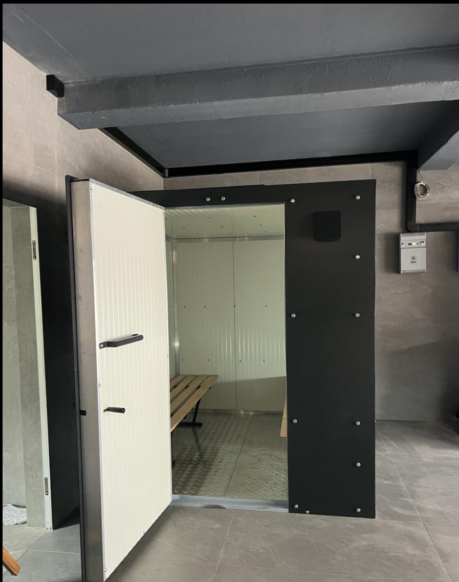
Shelter interior showing integrated benches and heavy non-slip floorplate
